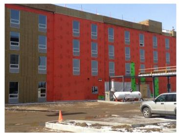
Over 2,787 m2 of WrapShield SA Self-Adhered Air Barrier (orange) was installed on the new "hip and humble" Home2 Suites.
