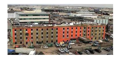
WrapShield SA Self-Adhered can be installed in temperatures as low as 20°F (-6°C) and can help to prevent weather delays.
