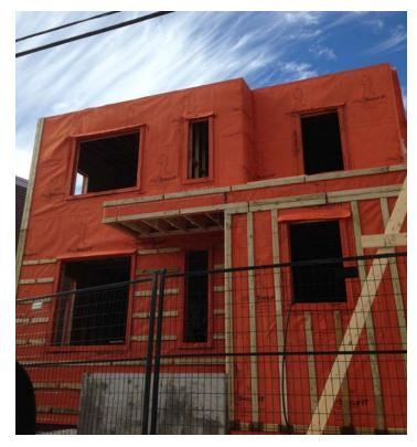
Over 3,000 sq. ft. (278.71 M²) of WrapShield Water Resistive Vapor Permeable Air Barrier Membrane was installed on this modern urban home located in Halifax, Nova Scotia.
