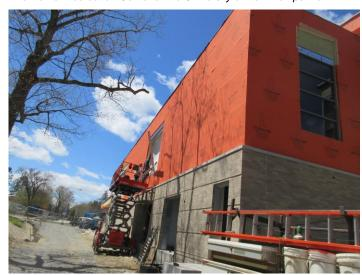
WrapShield SA Self-Adhered was chosen because its free of harmful VOCs and no primer is required, making it safe to install on campus.
