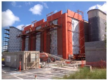
Over 16,000 sq.ft. of WrapShield SA Self-Adhered was installed on Horry Georgetown Technical College.
