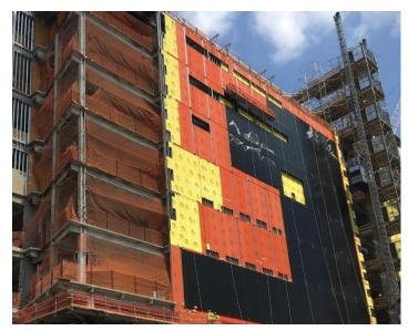
WrapShield SA Self-Adhered is phase construction friendly, can be installed in all weather conditions and sustains 180 days UV and climate exposure prior to cladding installation.
