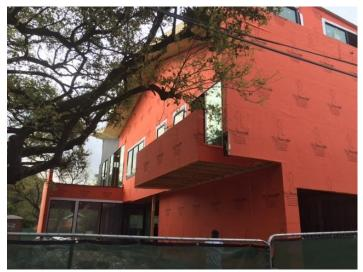
RevealShield SA Self-Adhered and WrapShield SA Self-Adhered do not require any substrate preparation, reducing labor costs.
