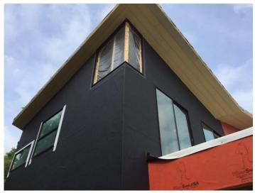
Over 8,000 sq.ft. of RevealShield SA Self-Adhered and WrapShield SA Self-Adhered were installed at the private residence in Houston.
