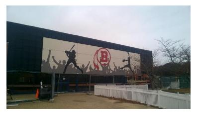
Approximately 2,500 sq. ft. of RevealShield UV Stable Water Resistive Vapor Permeable Air Barrier Membrane was installed on Barnstable High School behind Fundermax panels.
