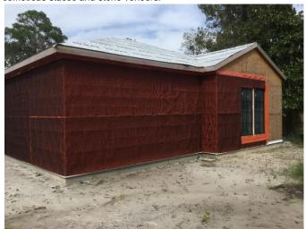
WrapShield RS Rain Screen was installed over multiple substrates including plywood and ICF (Insulating concrete form) and behind stucco and stone cladding..
