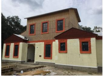
WrapShield RS Rain Screen offers an all-in-one weather resistive barrier, air barrier and 7mm rain screen drainage matrix, helping to dry out cemetious stucco and stone veneers.
