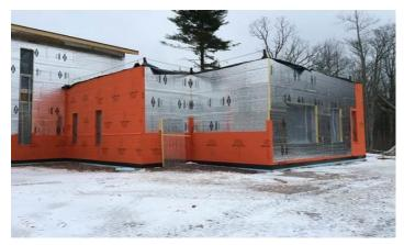
The Bear Creek Community Charter School in Pennsylvania was installed with roughly over 30,000 sq. ft. of WrapShield SA Self-Adhered Water Resistive Vapor Permeable Air Barrier Membrane, which was adhered to Dow Thermas™ Foil Faced Polyiso Sheathing.
