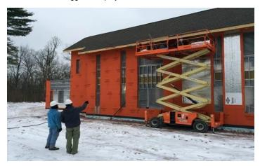
Even since the project's inception in January 2015, WrapShield SA Self-Adhered proved to withstand exposure to nature's harshest elements well into the spring season without faltering.
