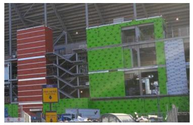
Over 50,000 sq. ft. of WrapShield SA Self-Adhered Water Resistive Vapor Permeable Air Barrier Sheet was installed on the renovated BMO Field in Toronto. Ontario in Canada.
