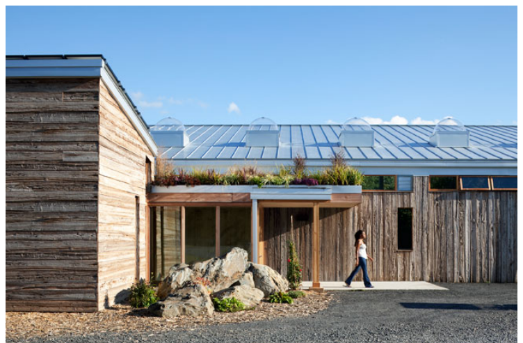
The Omega Institute is powered by a 48.5 kW solar electric system and also houses a water reclamation facility for wastewater filtration and treatment.
