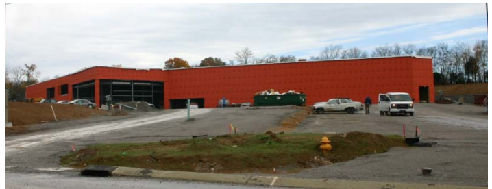
Installation complete for WrapShield (orange)
