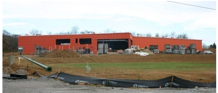
Installation complete for WrapShield (orange)
