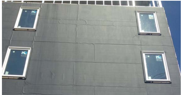
Over 120,000 sq. ft. (11,148 M 2 ) of RevealShield SA Self-Adhered is installed on Avonhurst Gardens in Dartmouth, Nova Scotia.
