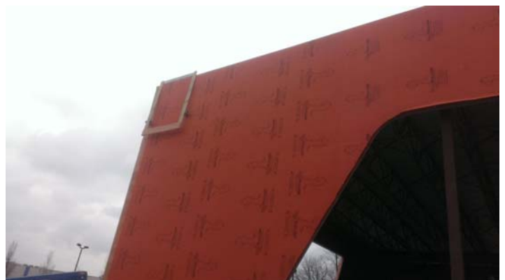
Offering multiple substrate compatibility, WrapShield SA Self-Adhered was installed over CDX plywood.
