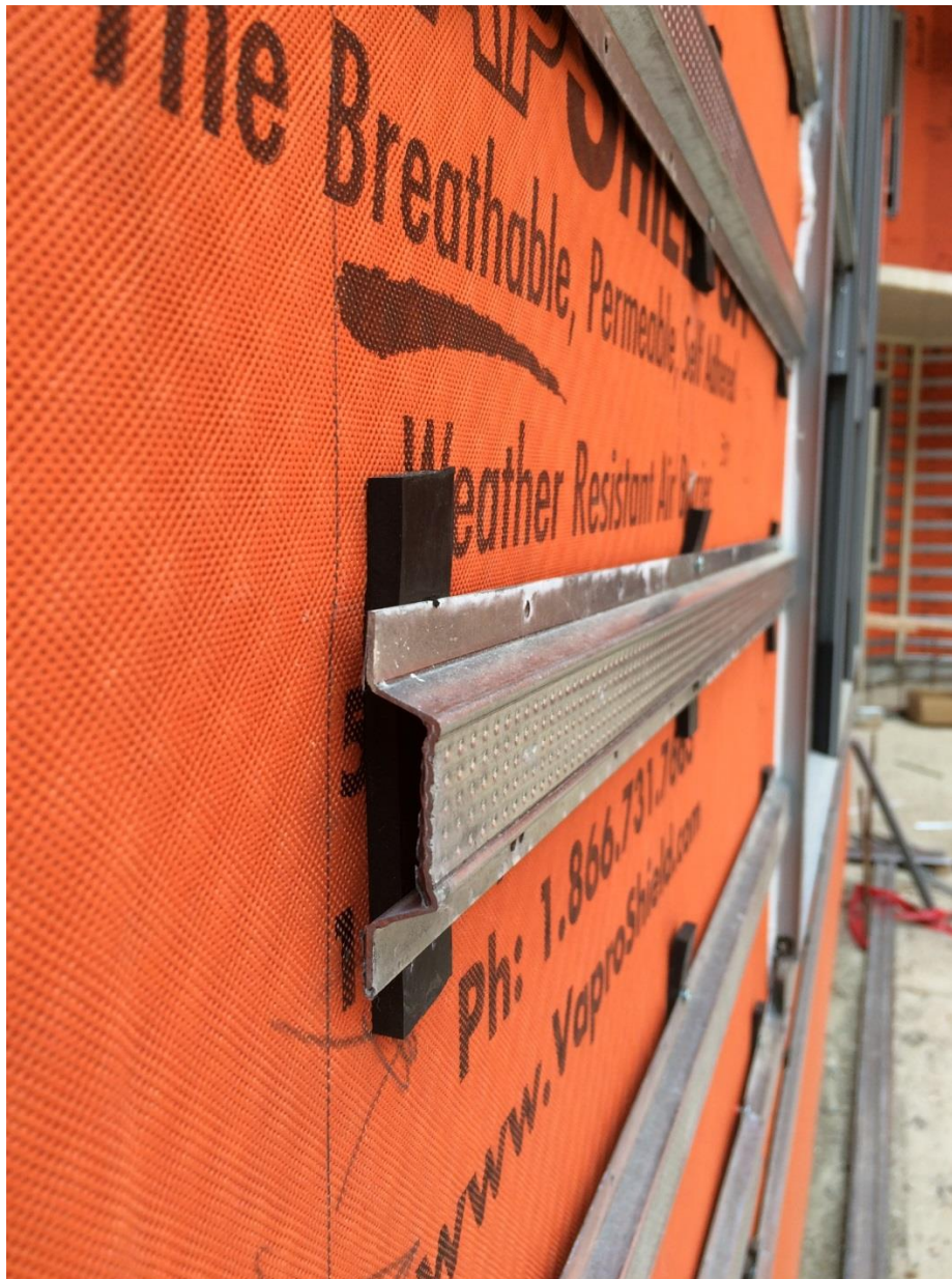
VaproShims used under horizontal cladding attachment created a small, effective ¼" rain screen cavity, allowing for unimpeded vertical drainage of moisture away from the building envelope.
