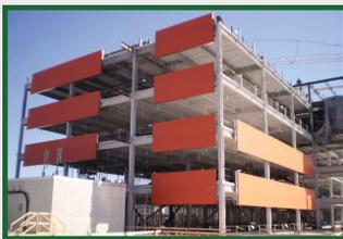
VaproShield WrapShield SA Self-Adhered membrane was installed in the \$150 million expansion of the Central Washington Hospital. Over 60,000 Sq.Ft. of membrane was used for complete adhesion to the modular wall system, protecting the panels during shipping and while exposed during construction.
