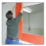
6. Install left & right jamb flashing, adhering the entire flashing to the left and right of the jamb by removing the release paper starting at the top and slowly pulling down, smoothing with your other hand as you remove the release paper.
