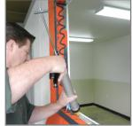
12. Apply additional VaproLiqui-Flash in zigzag pattern on all inner surfaces of the rough opening.
