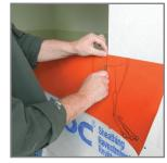
4. Slit material at corners to allow it to fold into the opening.
