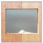
Before beginning, make sure all sheathing materials are clean, free of dust, and trimmed flush with framing members at rough openings and that all materials, sausage gun, and putty knife are on site.
