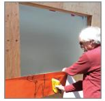
2. Install flashing at sill by minimally stapling it to the sheathing, leaving the lower 6" free for shingling over wall membrane.
