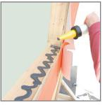
6. Using the sausage gun, apply VaproLiqui-Flash in a zigzag pattern on outer 2.75" of inside of rough opening.
