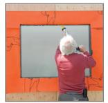
8. Using the sausage gun, apply a second layer of VaproLiqui-Flash over the folded flaps in a zigzag pattern on the inner surface of the rough opening.
