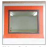
11. Immediately spread the applied material with a putty knife creating a 1" border around the rough opening.
