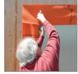
5. Slit each piece where it meets rough opening corners to allow center 2.75" deep flap to fold into the opening.
