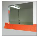
5. Fold flap into opening and adhere to inside surface, being sure to keep the lower 6" of release paper intact.
