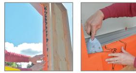
7. Immediately fold flaps into opening, pressing into the VaproLiqui-Flash with putty knife, spreading VaproLiqui-Flash evenly beneath VaproFlashing.
