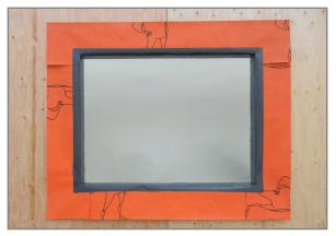
12. Allow VaproLiqui-Flash to set up until dry to the touch, then inspect for voids and apply additional VaproLiqui-Flash as needed to achieve complete coverage.
