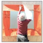
4. Install head flashing after left & right jamb pieces.
