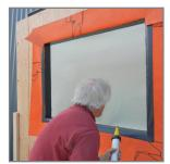
10. Apply VaproLiqui-Flash in a zigzag pattern on the wall face surrounding the rough opening.
