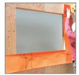
3. Install left & right jamb flashing with minimal stapling, allowing for later shingling with wall membrane.
