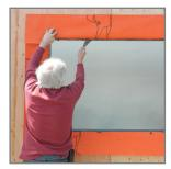
9. Immediately spread the applied material with a putty knife, fully embedding the inner flaps of VaproFlashing sill, right & left jamb, and head pieces, fully covering all inner surfaces of rough opening.
