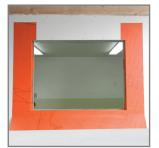
8. Install head flashing only after both left & right jamb pieces are fully adhered.
