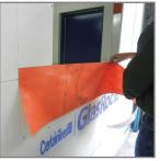
3. Install VaproFlashing SA at bottom of sill by removing release paper from top 6" of flashing material and sticking it in place, leaving 6" of release paper on the lower half of the material for shingling over membrane.
