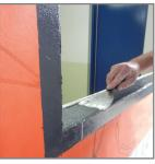
14. Allow VaproLiqui-Flash to set up until dry to the touch, then inspect for voids and apply additional VaproLiqui-Flash as needed to achieve complete coverage.
