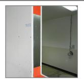
1. Cut and install VaproFlashing SA patches over pre-punched holes in metal studs, if present.
