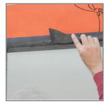
11. Immediately spread the VaproLiqui-Flash with a putty knife creating a 1" border around the rough opening (approximately 12 to 15 wet mils), paying special attention to the corners and edges.
