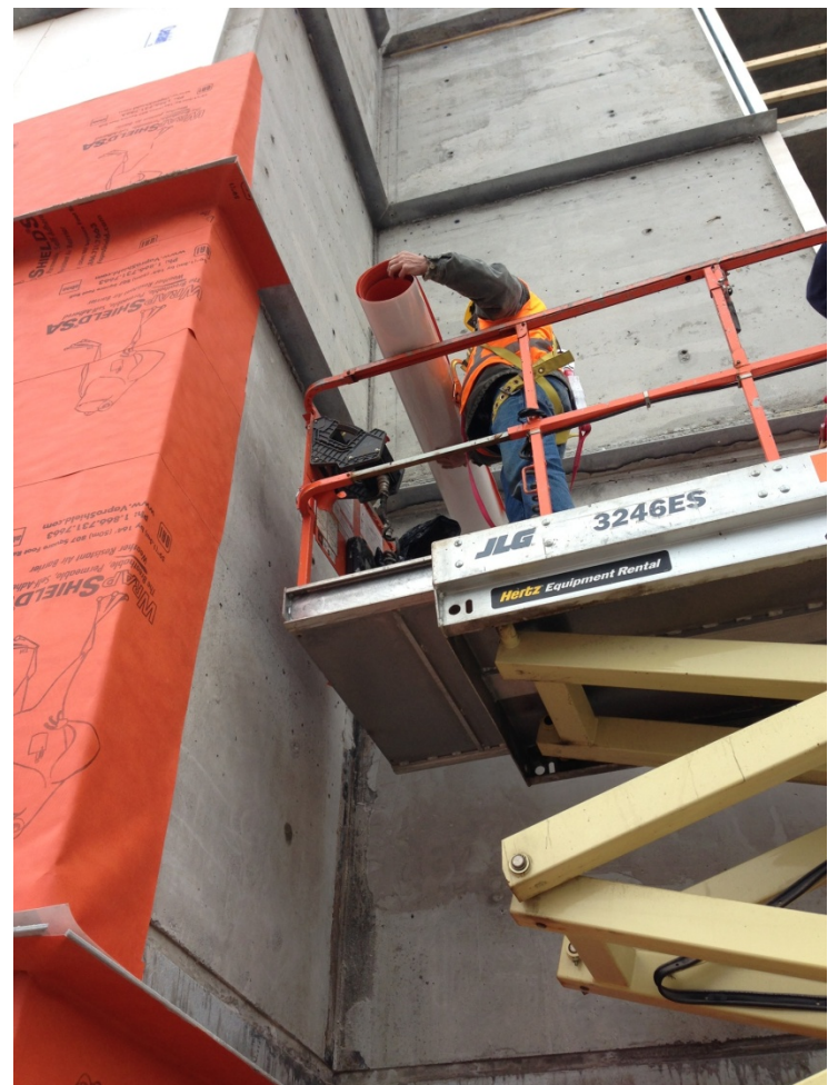
WrapShield SA Self-Adhered was adhered to both GlasRoc ® sheathing and concrete.
