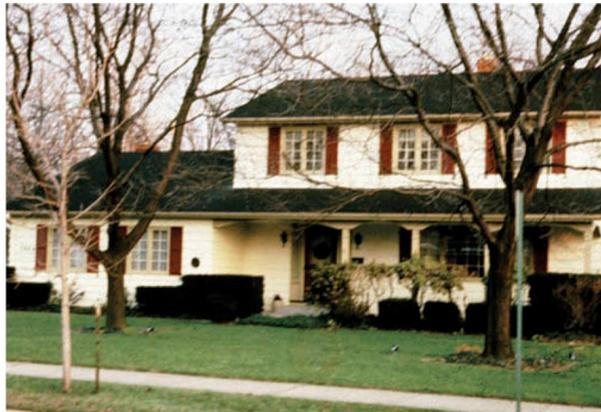
**Photograph 1: The “Typical House”**—Built in 1965 in Cleveland, OH with no cavity insulation in the exterior wood frame walls. No problems for twenty years. Insulation added to exterior walls in 1985 and within one year the paint begins to fail.
