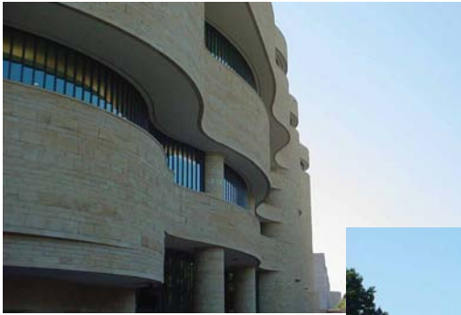
The National Museum of the American Indian (NMAI) is a new Smithsonian Museum in Washington, DC. The Smith Group was the architect for the building, using a Blueskin SA sheet membrane air/vapor barrier with BASF Walltite sprayed polyurethane foam insulation behind sandstone.
