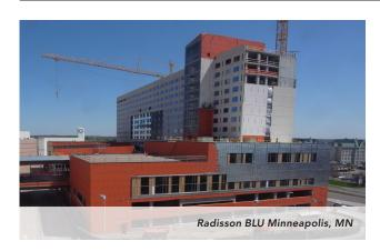
WrapShield SA Self-Adhered was successfully installed without any construction delays during the harsh Minnesota winter. The average temperature was between 10–30°F (-12–-1°C) with frequent high winds.
