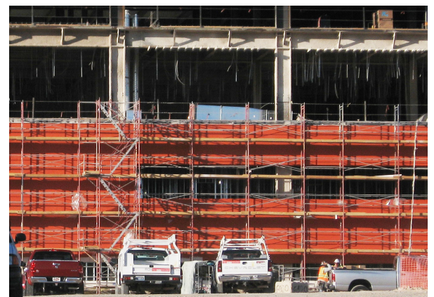
Veteran's Administration Main Hospital, North Las Vegas, NV 300,000 Sq. Ft. of WrapShield SA Self-Adhered with Trespa, metal and brick exterior cladding.
