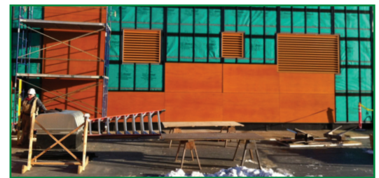
WallShield, a high-end weather barrier, allows any consequential moisture in the wall system to breathe out, as seen on the Covenant House in Anchorage, Alaska.
