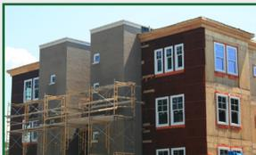
Over 250,000 sq. ft. of WrapShield HS Water Resistive Vapor Permeable Air Barrier Sheet with Drainage Matrix was installed on nine College Town student housing buildings in Ithaca, NY.
