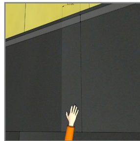
6. Lay overlapping layer of RevealShield onto vertical sealant joint and smooth with hand pressure.
