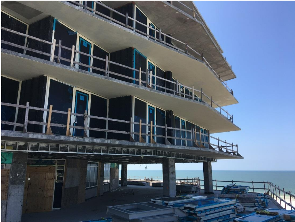
65,000 square feet of RevealShield SA Self-Adhered (black) withstood the forces of Hurricane Irma
