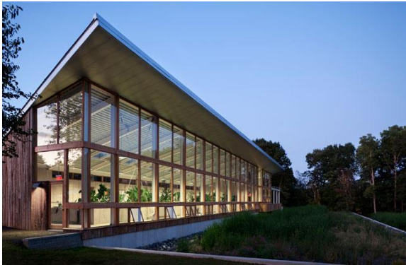
Omega Institute for Holistic Studies trusted VaproShield's membranes to meet the Living Building Challenge's rigorous standards. Photo courtesy of Green Source.
