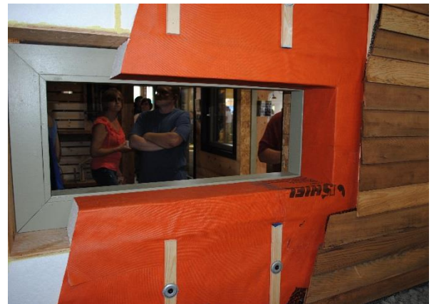
North Dakota State U Passivhaus uses very little energy for heating and cooling costs with its airtight building envelope using VaproShield WrapShield SA® Self-Adhered.
