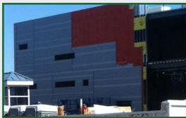
Over 65,000 sq.ft. of WrapShield SA Self-Adhered Water Resistive Vapor Permeable Air Barrier Sheet was installed on the Pier 27 Cruise Terminal in San Francisco. The terminal is to include a year-round cruise terminal, public plaza, and community facility. With the award of the America's Cup to San Francisco, the pier will also be used as the starting and finishing line for the race in 2013.
