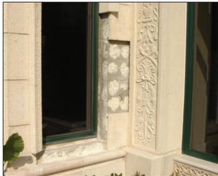
**Photo 5:** Precast Elements. “Mud-set” precast elements installed over the top of direct applied stucco.
