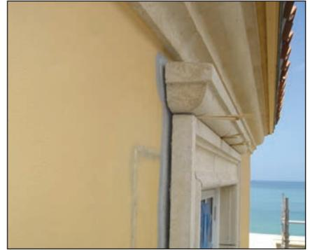
**Photo 2:** Gap Behind Siding and Trim. With wood and fiber cement siding and trim, you need to install the siding and trim over a small gap to control hydrostatic pressure. This gap can be as small as 0.25 in. and the spacer can be a strip of thin foam.
