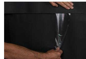
Peel back release films to finish horizontal seam. For complete installation instructions, visit [VaproShield.com](http://VaproShield.com).
