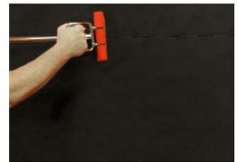
Roll the integrated tape seam with floor roller to ensure full contact
