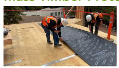
Install SlopeShield Plus SA over mass timber roof deck/floor deck to protect it from moisture intrusion and construction damage. See separate product data sheet at VaproShield.com.
