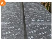
Install SlopeShield Plus SA over mass timber roof deck/ floor deck to protect it from moisture intrusion and construction damage. Tape all seams using VaproTape.
