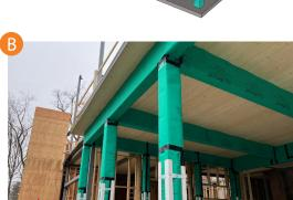
Wrap post/columns and beams with WallShield IT to protect against moisture intrusion and construction damage. Use aproTape to hold seams together when required.
