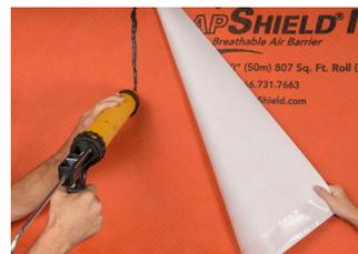
Overlap vertical seams by min. 12". Apply 1/4" (6.4 mm) bead of VaproBond adhesive sealant to ensure water and
