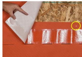
Secure membrane with stainless steel staples **above** integrated tape. Align the bottom of the upper course with the dotted line for proper 6" (15 cm) overlap.
