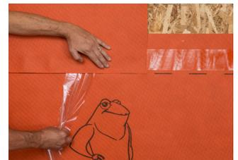
Join horizontal seams by peeling back both release films. Tape seals horizontal seams.
