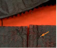
3. Mechanically fasten Vapromat approx. 2" down from the top edge with stainless steel (SS) staples.
