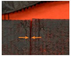
4. Vertical seams of VaproMat drainage matrix butt together and do not overlap.
