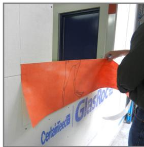
3. Install WrapFlashing SA at bottom of sill by removing release paper from top 6" of flashing material and sticking it in place, leaving 6" of release paper on the lower half of the material for shingling over membrane.
