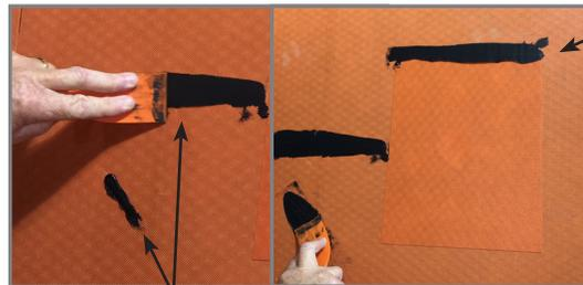
**Abrasion Repair:** apply VaproBond over abrasion and tool with a DRY joint knife, trowel or spatula.
