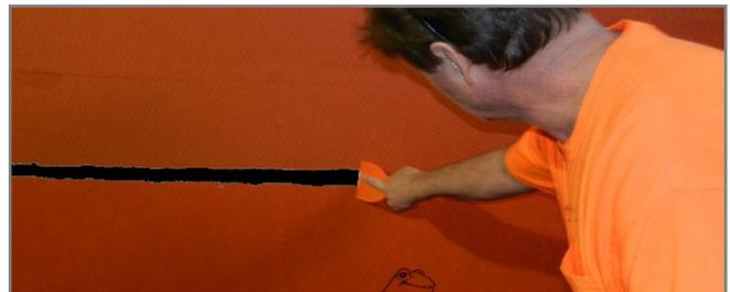
Use a DRY joint knife or trowel to tool VaproBond to shed water.
