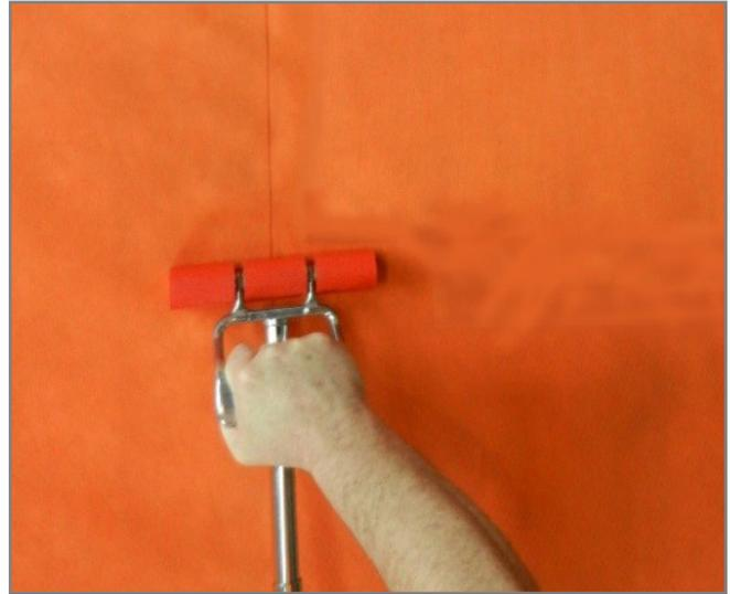
Use hand roller to seal the seam for an air and water tight seal.
