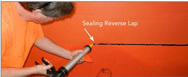
Apply 3/8" (9.5mm) minimum bead line of VaproBond to the reverse lapped membrane.
