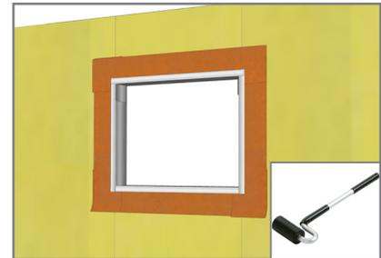
6. Install Vapro-SS Flashing on head in shingle fashion with 3" up-turned legs at sill and head + 1" on face; jambs are 1" onto the face. Roll all Vapro-SS Flashing with weighted roller to ensure full contact.
