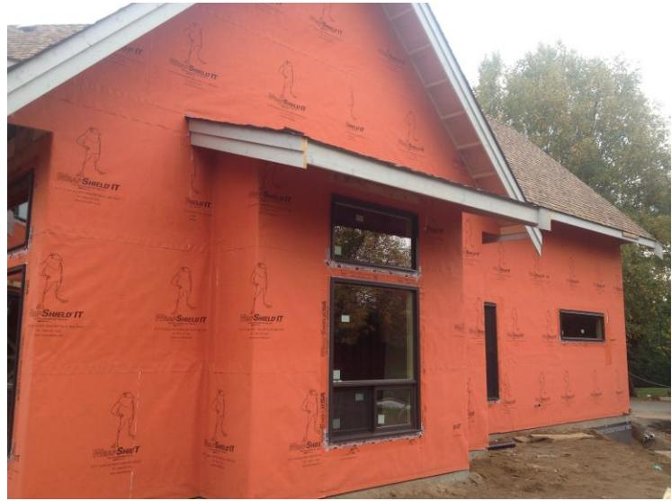
Over 4,000 sq. ft. (1,219 M<sup>2</sup>) of WrapShield and WrapShield SA Self-Adhered Air Barrier is installed on a private residence in Langley, British Columbia.
