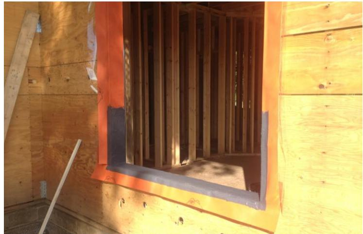
(above) VaproLiqui-Flash (gray) liquid applied waterproof flashing material is applied around the rough opening of a window.
