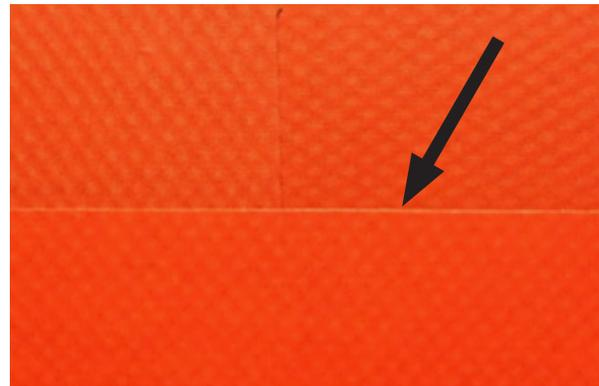
*Figure 2, On the upper reverse lap seam, apply a bead of VaproBond™ sealant the full length of the seam, as shown in Figure 3*
