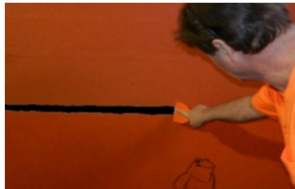
*Figure 4, Feather the bead of VaproBond™ using a hand trowel*
