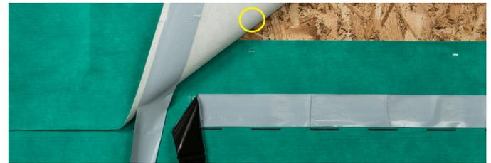
Secure membrane with stainless steel staples above integrated tape. Align the bottom of the upper course with the dotted line for proper 6" (15 cm) overlap.
