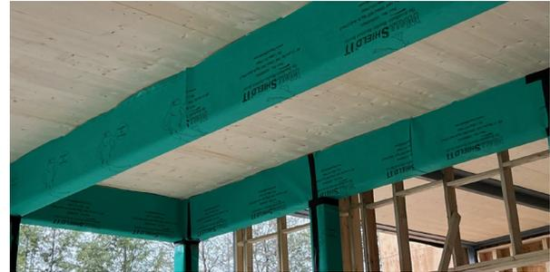
With a drying capacity of 123 perms, the framework dries out quickly and is less susceptible to ongoing wetting issues from weather events.
