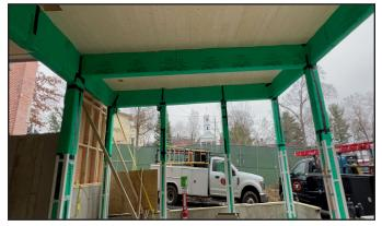
2. Wrap post/columns with WallShield IT to protect against moisture, mold, and construction damage. Use VaproTape to hold seams together when required, add corner protection (by others).
