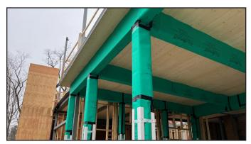
4. Connect and/or install wrapped post/column to wrapped beam. Use VaproTape as required on seams.
