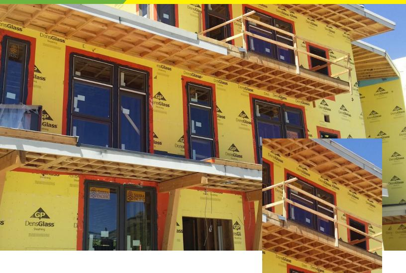
Over 20,000 sq. ft. of WrapShield SA Self-Adhered was installed on the Lot 4 LUMIN residences at Snowmass Base Village in Snowmass, Colorado.
