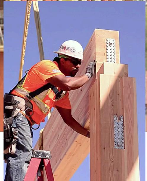
40,000 sq. ft of WrapShield SA Self-Adhered was installed on First Tech Credit Union, the largest documented U.S. building to use cross-laminated timber (CLT). The 156,000-square-foot building consists of glulam beams and CLT with a steel brace frame lateral restraint system.
