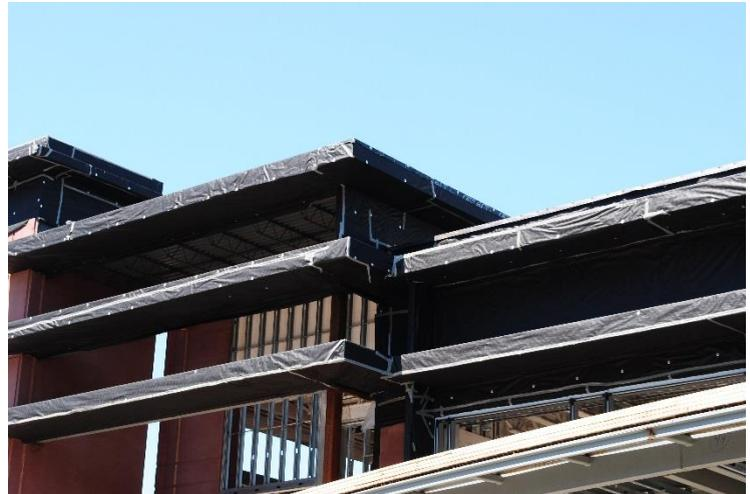
Over 40,000 sq.ft. of WrapShield Black Water Resistive Vapor Permeable Air Barrier Membrane was installed on the St. Cloud Civic Center.
