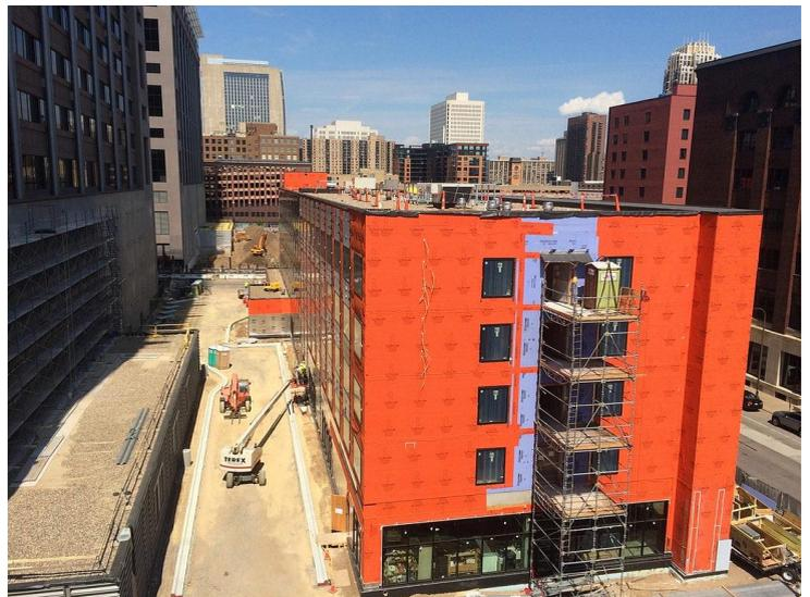
*WrapShield SA Self-Adhered withstands low temperature application and can be exposed for up to six months before cladding installation.*
