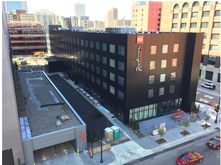
*WrapShield SA Self-Adhered was installed behind aluminum panels on the new Radisson Red hotel in Minneapolis, MN.*
