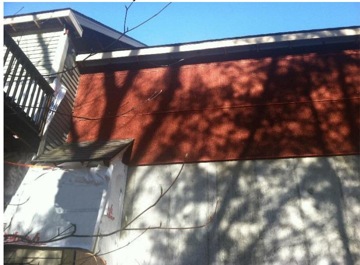
*WrapShield HS drainage matrix allows moisture to escape quickly while protecting the sidewall from the damaging effects of mold, mildew and moisture intrusion.*
