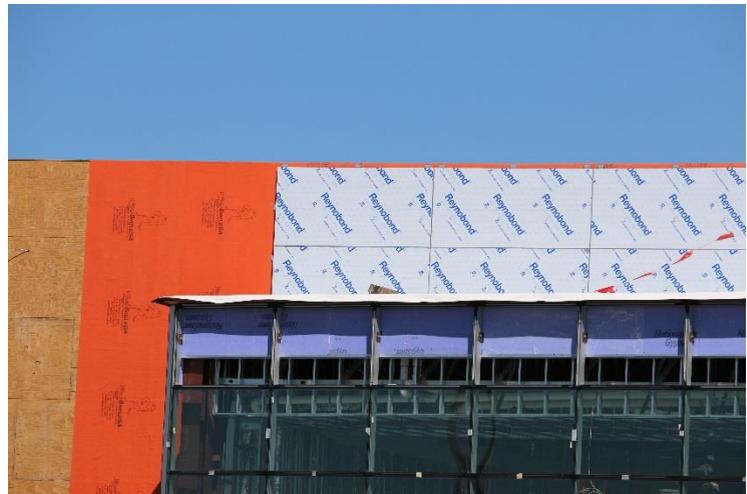
Multiple cladding types are being installed on this project including aluminum composite panels.
