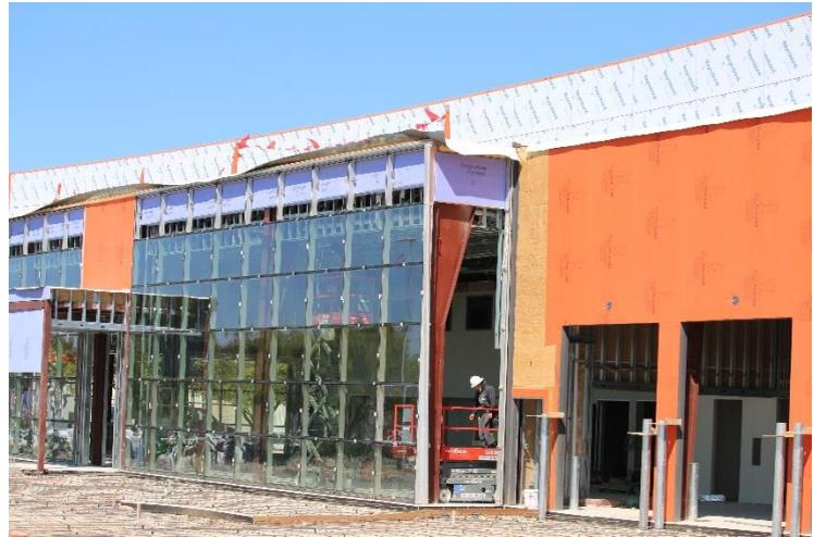
Over 15,000 sq.ft. of WrapShield SA Self-Adhered was installed over plywood on the new Ford dealership.
