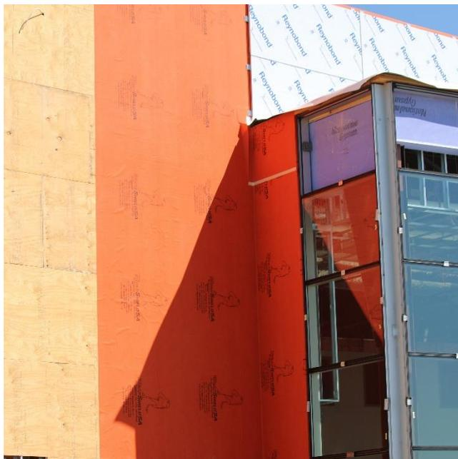
WrapShield SA Self-Adhered installed over plywood and behind aluminum composite panels.
