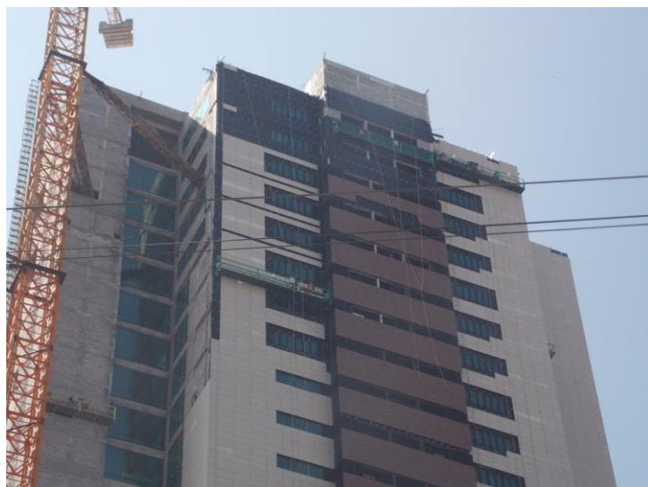
*RevealShield IT Integrated Tape applied directly to the large cement tower, helping to dry out the cementitious substrate.*
