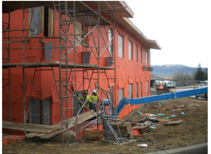
*WrapShield SA Self-Adhered withstands low temperature application and helps to dry out CMU and plywood.*
