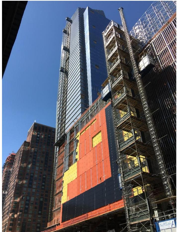
Over 40,000 sq.ft. of WrapShield SA Self-Adhered WRB/Air Barrier is being installed on Building #11 of the Hudson Yards Development in New York, New York.
